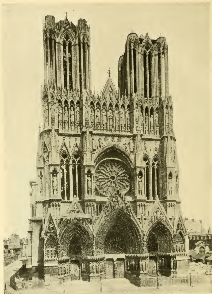
RHEIMS CATHEDRAL. — This supremely beautiful example of Gothic architecture (p. 304), dating back almost to the year 1200, was wantonly injured by German shells in the World War. Until 1100, the rather rude architecture of Western Europe was the Romanesque , based upon Roman remains and marked by the round arch and massive walls. The early architects knew no better way to carry the weight of immense stone roofs; nor did they dare weaken their gloomy walls even by cutting out large windows. In the 13th century, that Romanesque style was replaced by a new French style called Gothic . The architect, a better engineer now, had learned two new devices to carry his roofs. (See opposite.)
